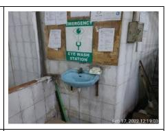
Eye wash station were found nonfunctional and without paddle push in the washing section NC Picture No. 06
